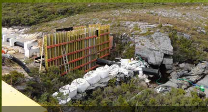
The work site showing the weir formwork in place and the temporary dam with the aggregate-filled fertiliser bags forming the bund.
