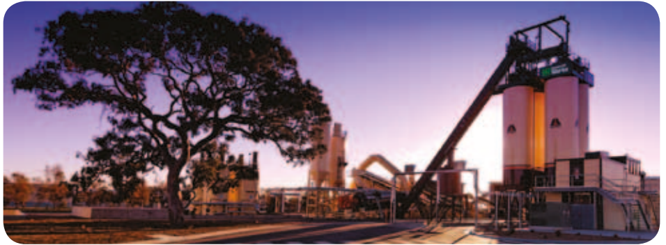
Downer's asphalt manufacturing plant at Sommerton, Victoria.
