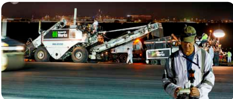
Downer Works wins NSCA award for innovative environmentally sustainable work practices.
